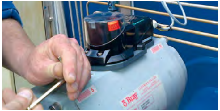
The F31K2 is easy to mount directly onto the pneumatic actuator. The sensor is directly attached to the drive housing, and the puck merely needs to be pushed onto the drive shaft and fixed in place according to the valve's current position.
