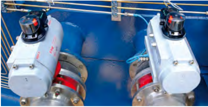
Two F31K2 dual inductive sensors mounted on pneumatic valve actuators at Frisia Zout in Harlingen, the Netherlands.
